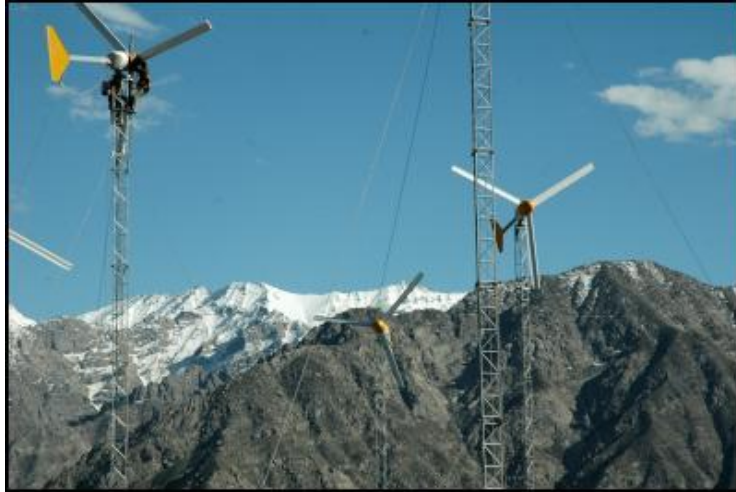
Afghanistan's first wind farm in Panjshir Province
